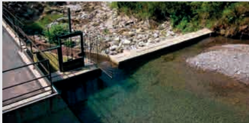
On the left: Lock in a water course reducing the flow downstream
